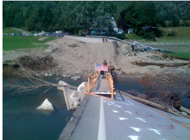
5 - Temporary footbridge over White River (Source: VTrans)
